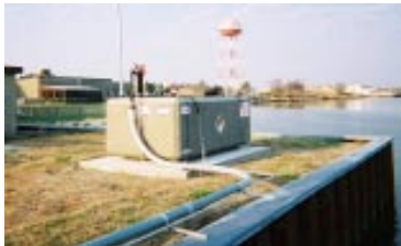
1000 Gallon ConVault w/ hurricane restraints
