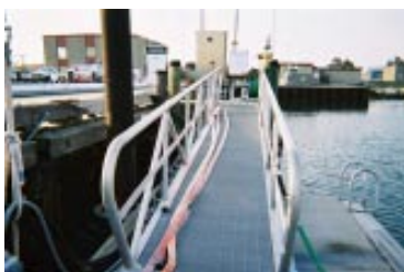
Custom made floating dock and pvc guide for hose
