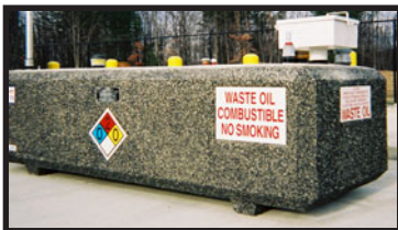
Waste Oil Disposal
